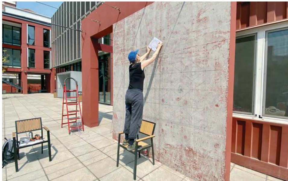
School helpers sand down the wall.
